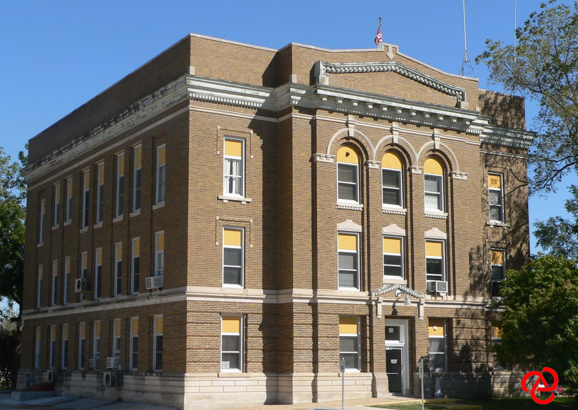
EXISTING COURTHOUSE – WEST FACADE
