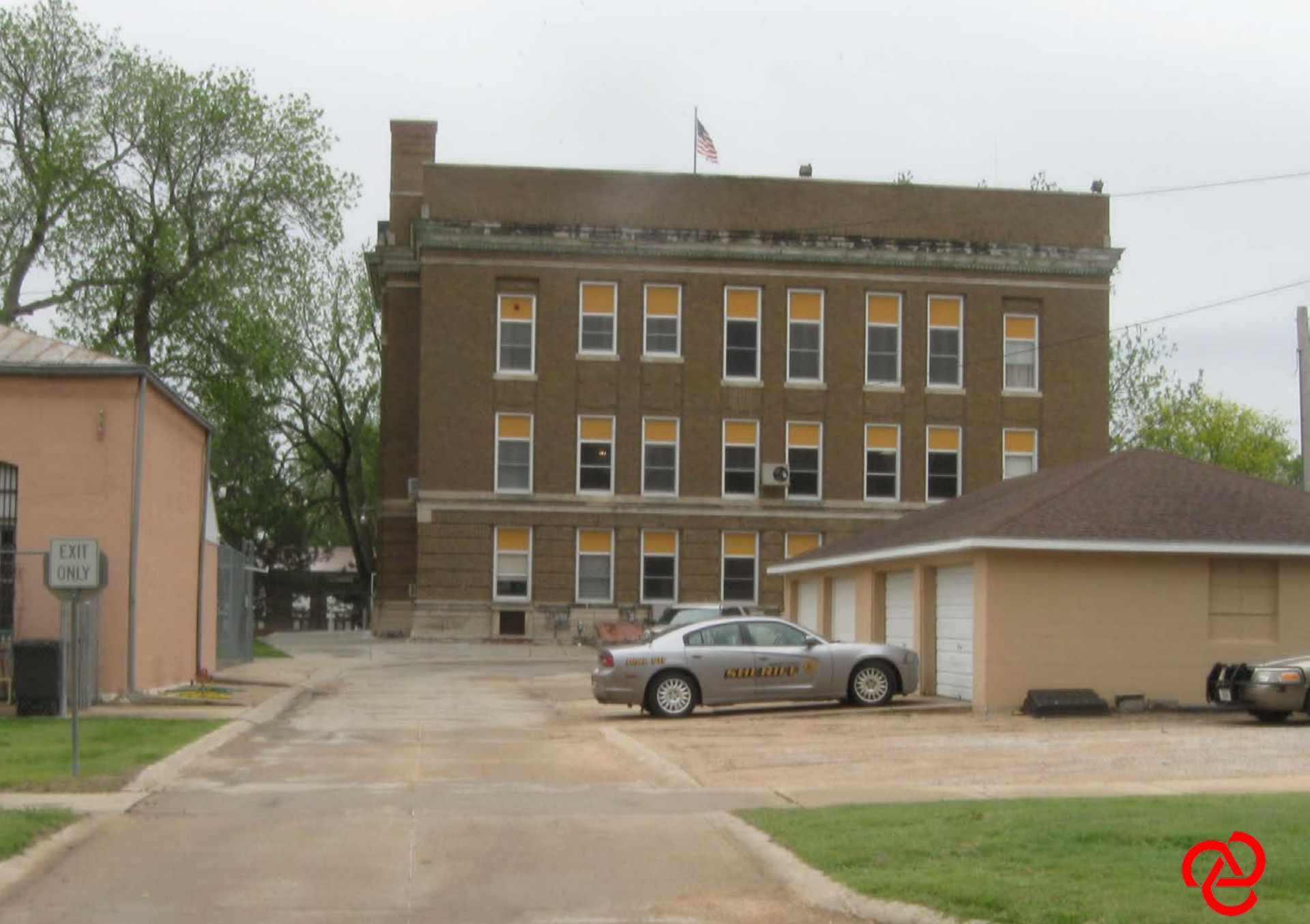
EXISTING COURTHOUSE – NORTH FACADE
