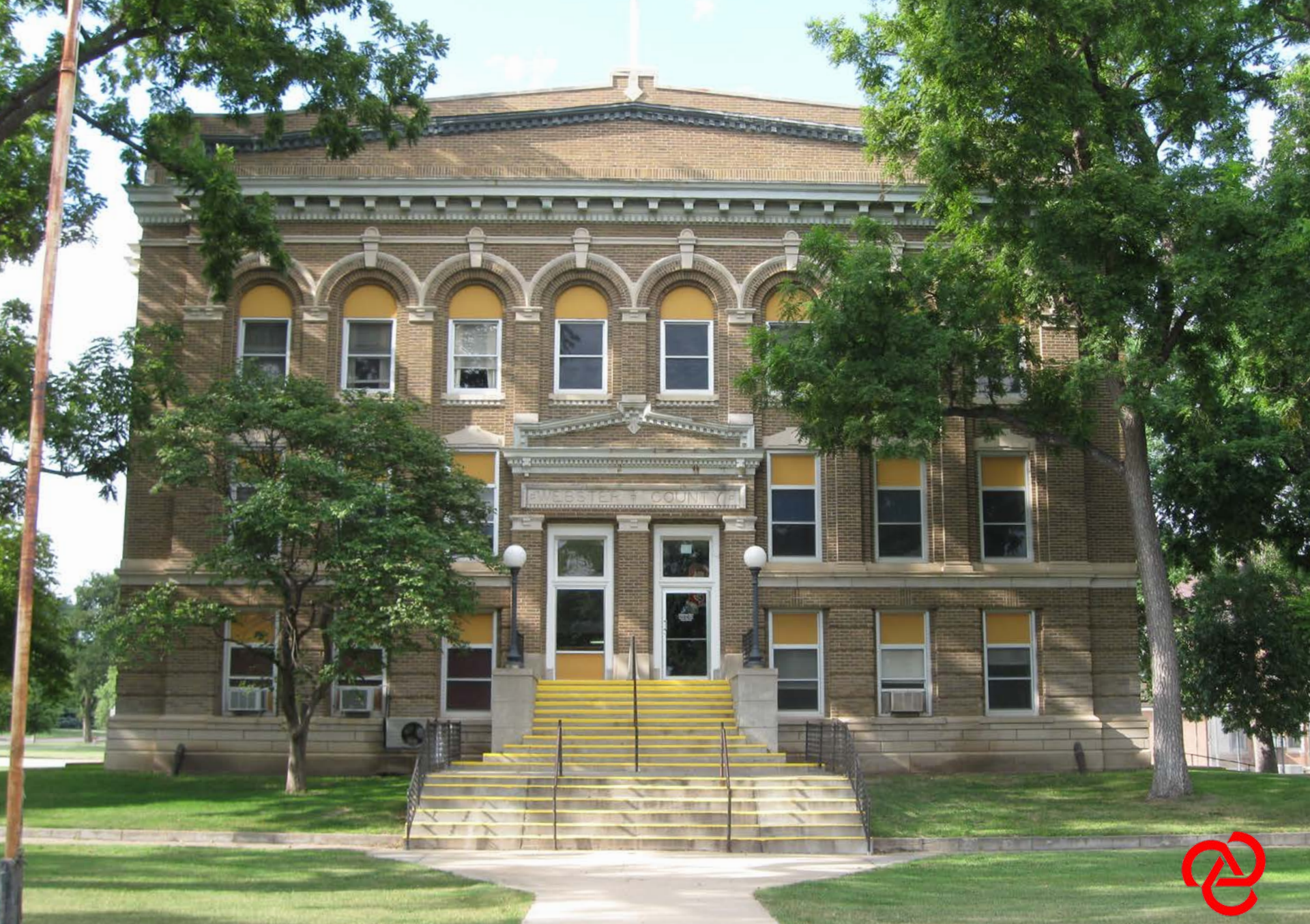
EXISTING COURTHOUSE – SOUTH FACADE
