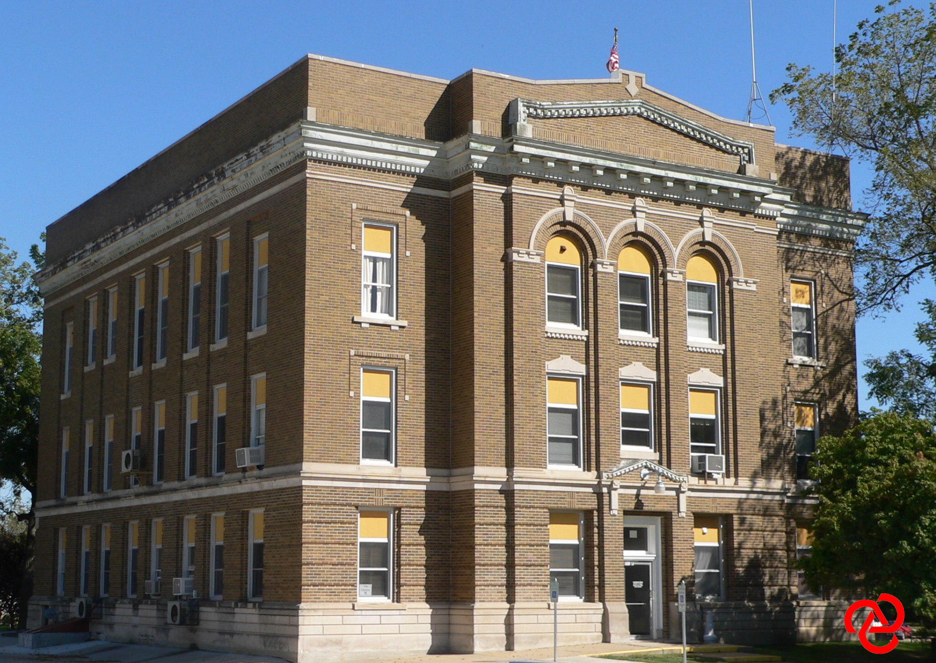
EXISTING COURTHOUSE – WEST FACADE
