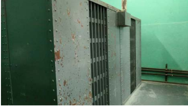
Figure 49 Prefab steel cell in open Day Room
