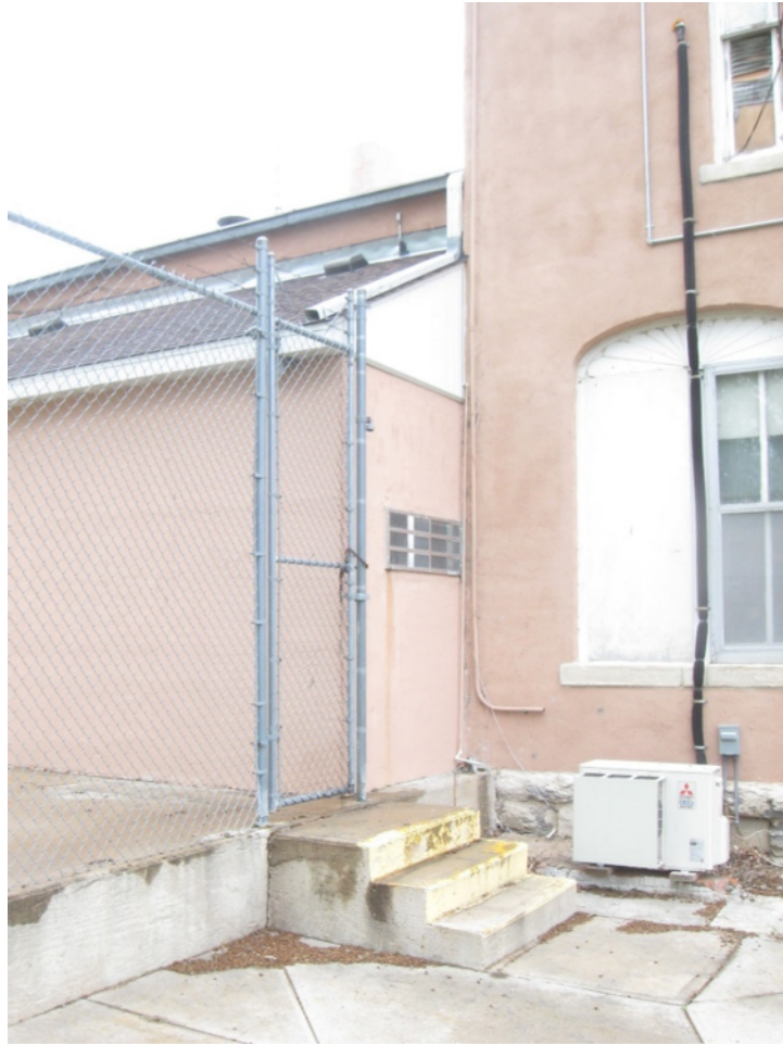
Figure 45 Southeast corner of addition and east side of Exercise area
