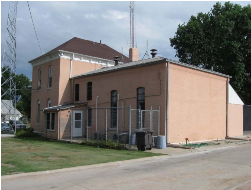
Figure 38 Jail Wing, facing northeast, showing delivery and staff entrance through the fencing
