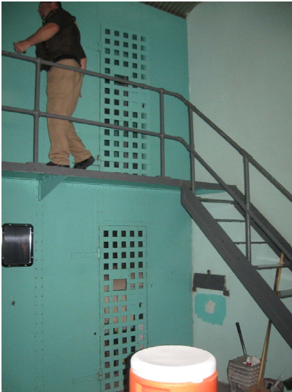
Figure 51 Prefabricated two-over-two steel cells
