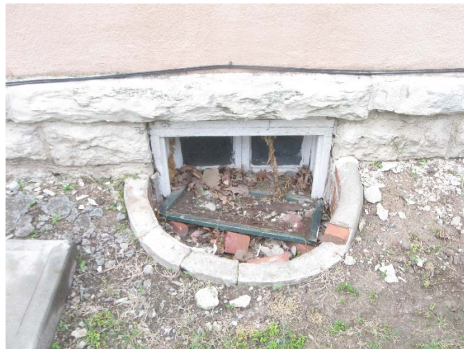
Figure 41 Typical basement window
