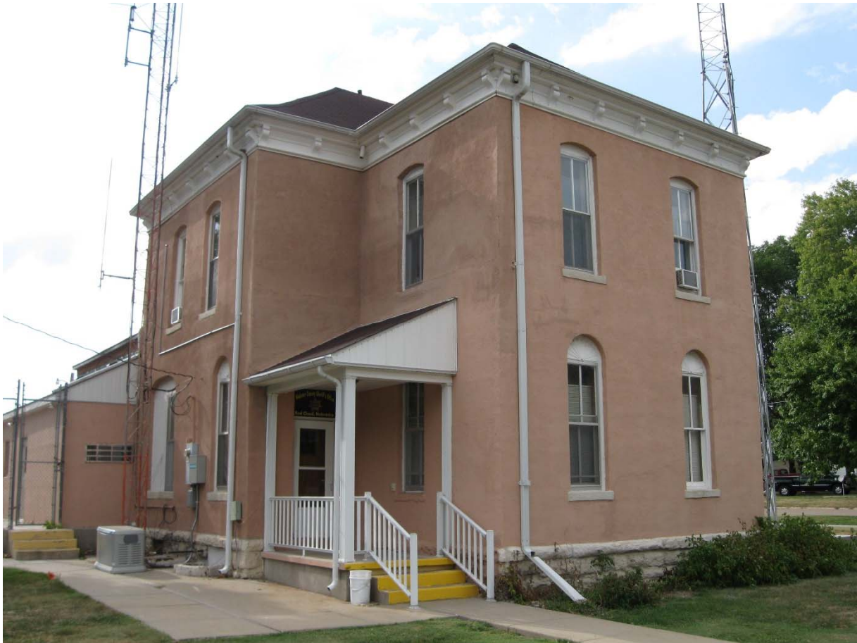
Figure 36 Entry façade, facing southeast.
