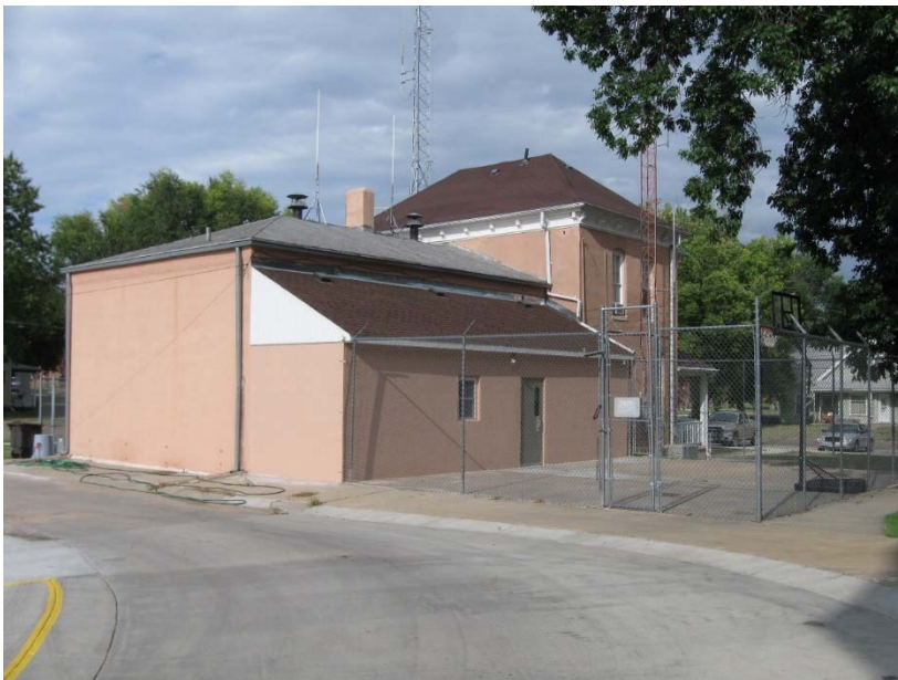
Figure 39 Jail Wing, facing southwest, with more recent lean-to addition.
