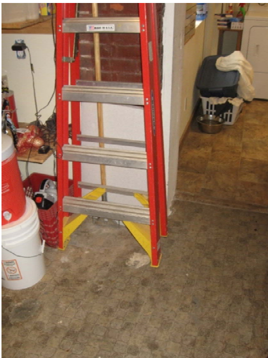
Figure 47 Interior floor of Pantry with step to Kitchen
