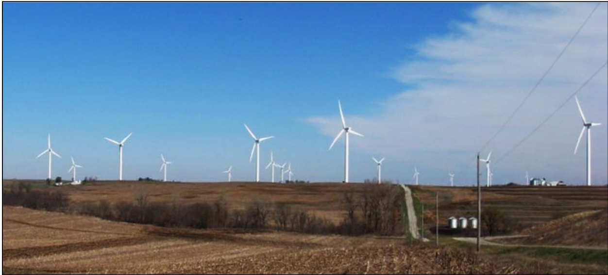
Steele Flats Commercial Wind Energy Conversion System in both Gage and Jefferson Counties.
